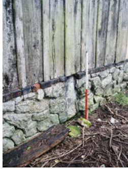
Ragstone dwarf wall supporting the existing building
