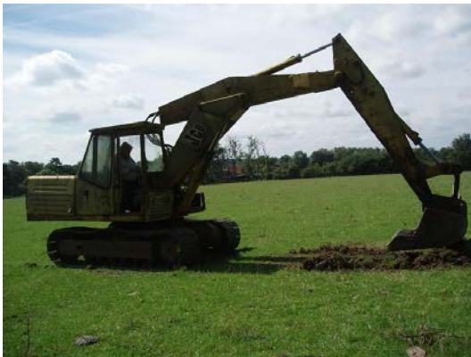
Digging the slot across the parch mark
