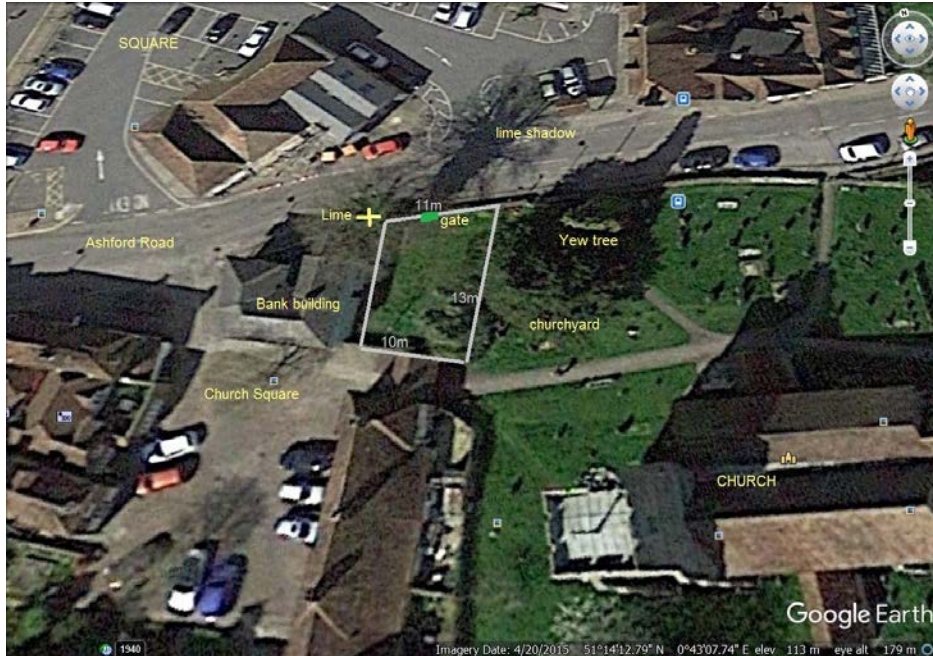
Google Earth view of the site 2015
